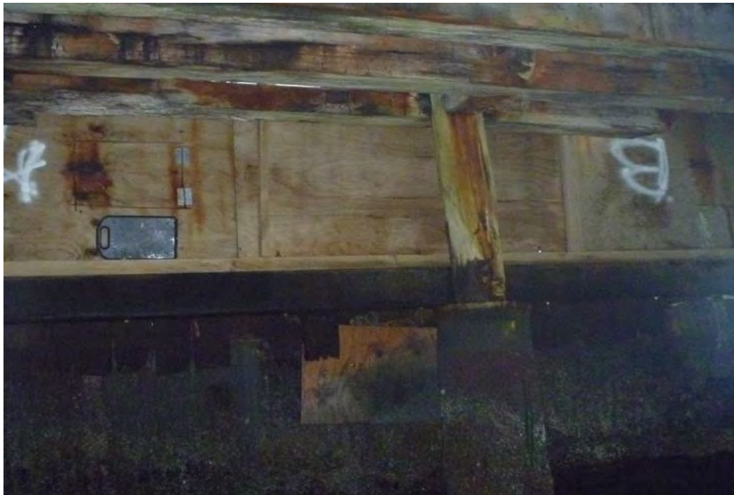
Photographs 5 & 6: Ply facing at Void A. Photographs above taken 22/06/2020. Photo below taken 10/10/2019.
