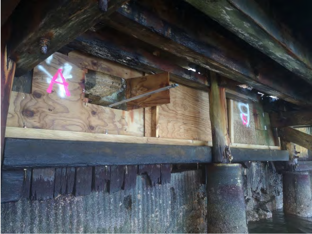
Photographs 5 & 6: Ply facing at Void A. Photographs above taken 22/06/2020. Photo below taken 10/10/2019.
