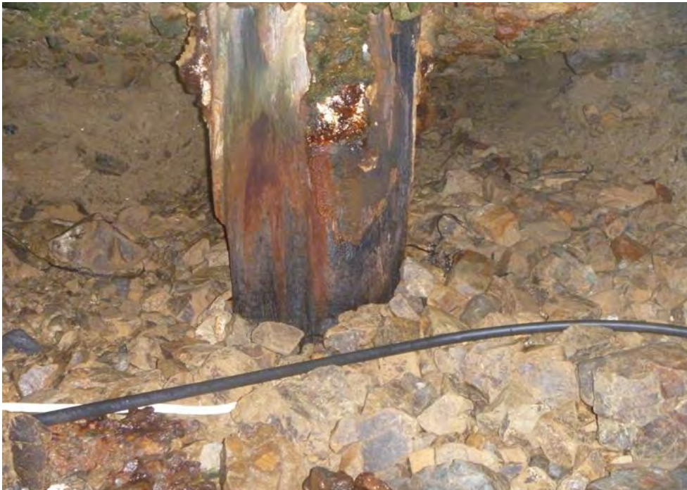
Photograph 13 & 14: Void C photo taken 22/06/2020 above. Below 10/10/2019. No noticeable further deterioration of pile nor erosion of void.
