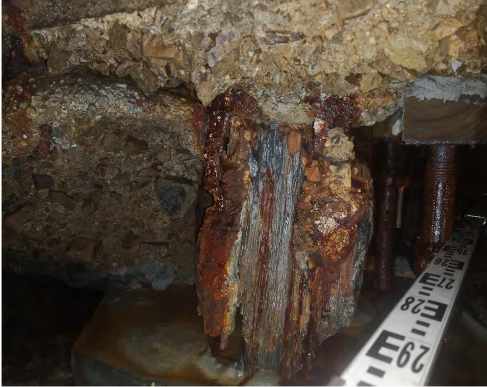
Photograph 9 & 10: Condition of temporary propping and grout pad in Void B. Photo 22/06/2020 above, 10/10/2019 below.
