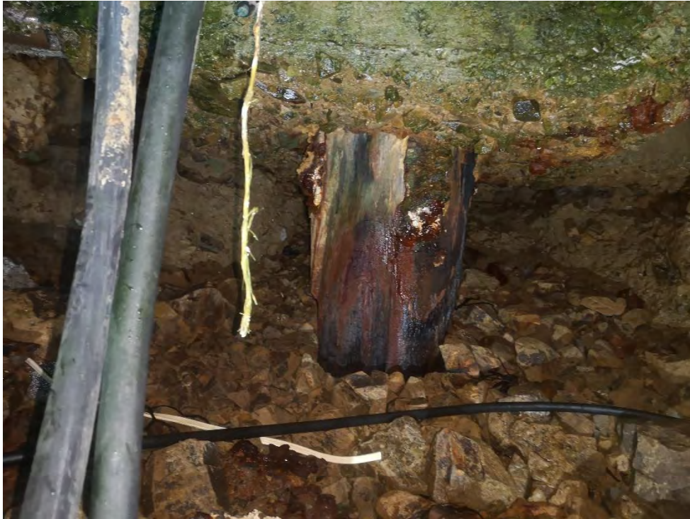
Photograph 13 & 14: Void C photo taken 22/06/2020 above. Below 10/10/2019. No noticeable further deterioration of pile nor erosion of void.
