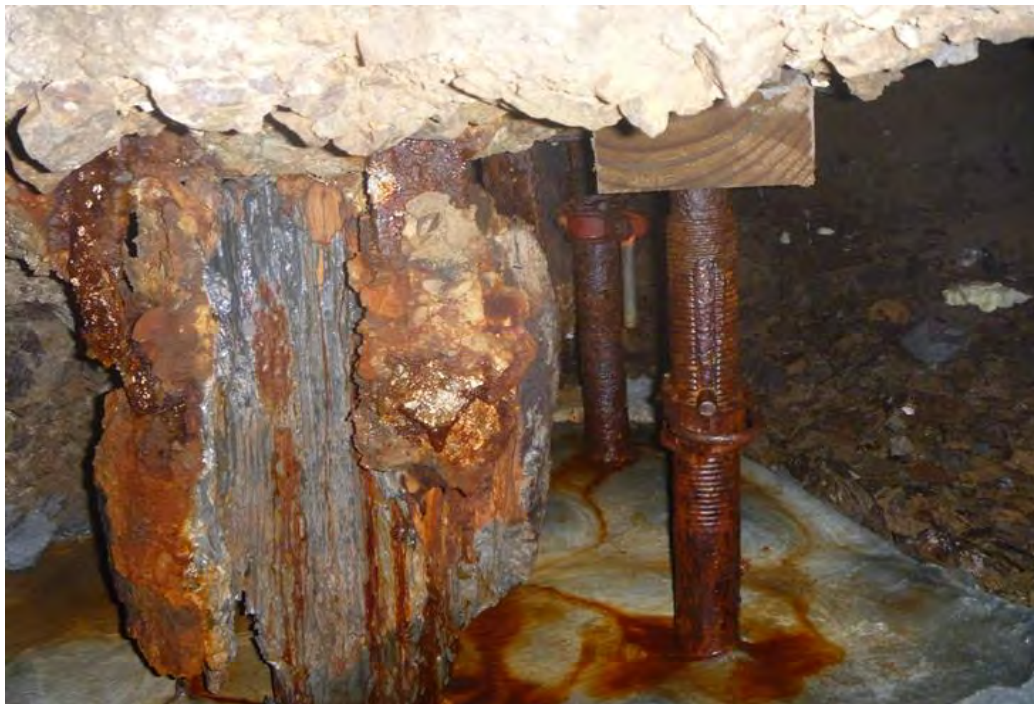
Photograph 9 & 10: Condition of temporary propping and grout pad in Void B. Photo 22/06/2020 above, 10/10/2019 below.
