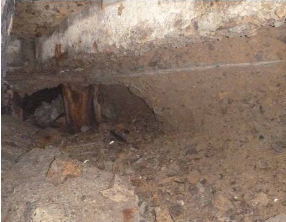
Photograph 17 & 18: Photo 17 above taken 09/03/2020 looking north from Void A. Condition of timber acceptable relative to other piles. Ply facing installed over damaged timber railings so no longer observable from Void D-South. Photo 18 below taken 10/10/2019
