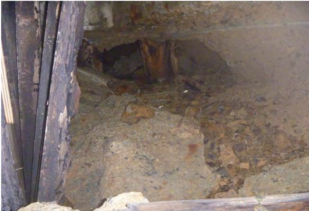
Photograph 17 & 18: Photo 17 above taken 09/03/2020 looking north from Void A. Condition of timber acceptable relative to other piles. Ply facing installed over damaged timber railings so no longer observable from Void D-South. Photo 18 below taken 10/10/2019
