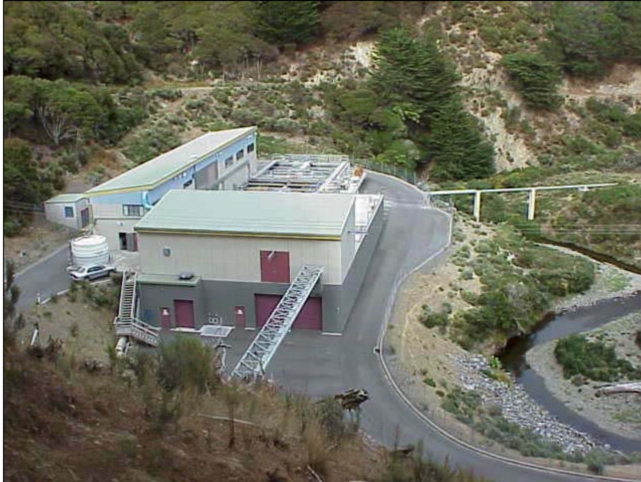
Western Wastewater Treatment Plant
