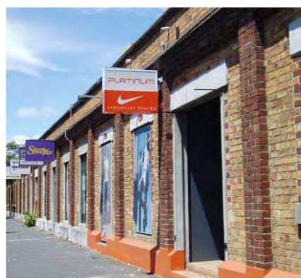
Example of projecting signs attached at right angles to the building façade
