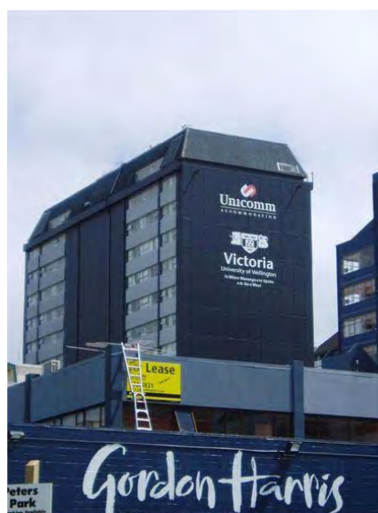
Example of signs painted on the building exterior
