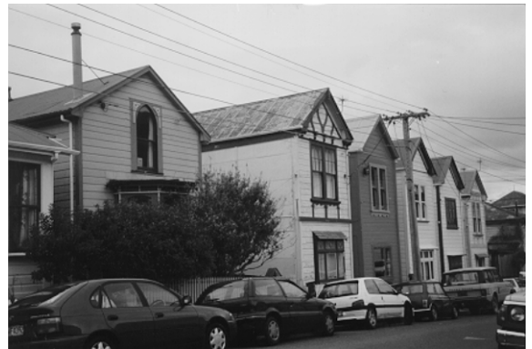
Notable concentration of identical double storey cottages on the western side of Porritt Avenue
