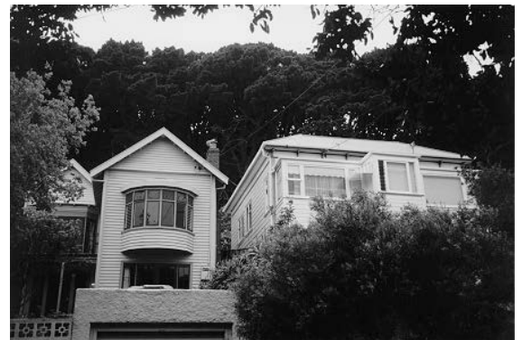
Double storey bungalows and villas are typical along the eastern, higher side of Scarborough Terrace
