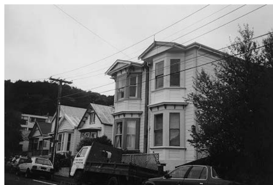
Pairs of terraced houses along the street
