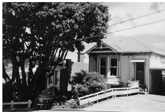
Single storey dwellings found along the western side of Hawker Street
