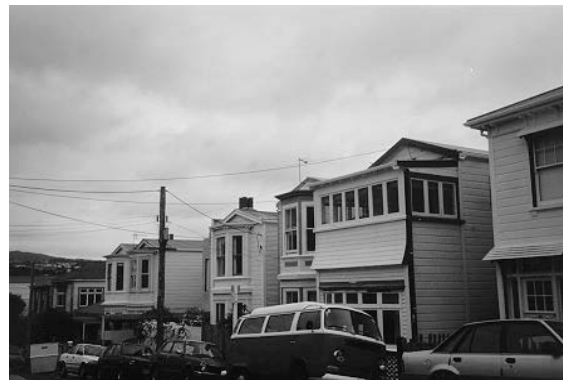
Consistent pattern of double storey dwellings along the northern side of Queen Street
