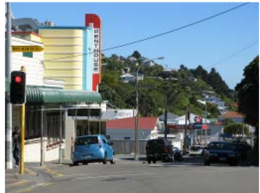
The prominent façade of the Penthouse Cinema is both a local landmark that signals an important community destination
