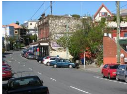
Gaps and variation in height and alignment along the street edge
