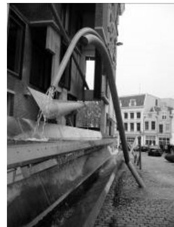
Richness of detail at ground level
