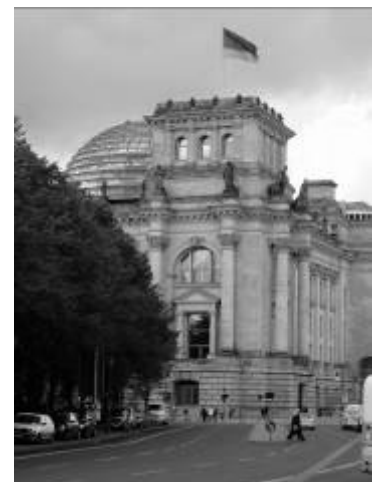
Publicly significant building demands contrast
