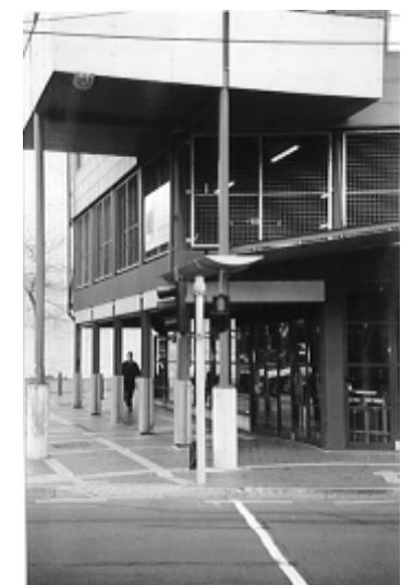
Building frontage to the street
