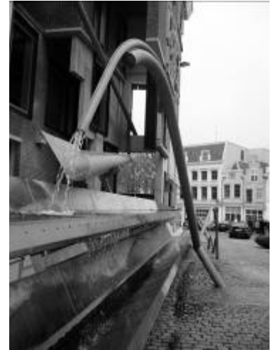
Richness of detail at ground level
