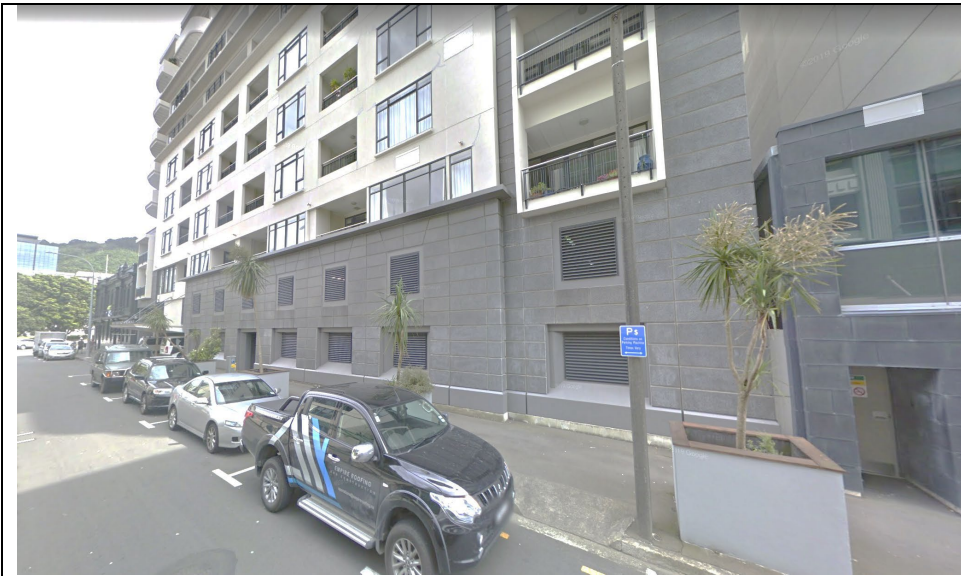
Figure 30 Kate Shepherd Apartments, Wellington, New Zealand. Trees planted by developer as alternative to a canopy wind shelter will never provide the promised shelter, and have become the responsibility of the City Council, not the building owner
