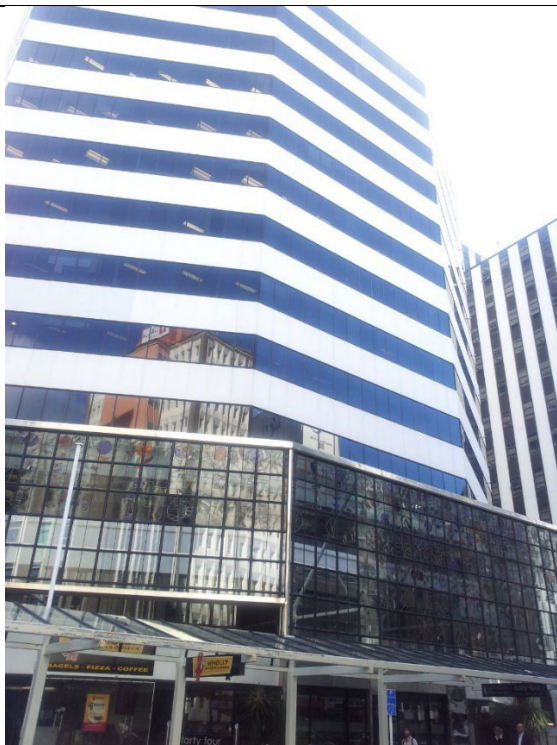
Figure 16 Aurora House, The Terrace, Wellington. This building has chamfered corners to reduce the width of the building 'catching' the wind; combined with a large glazed verandah
