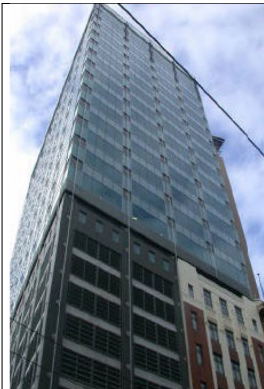
Figure 22 Example from Wellington of divided flows to reduce the problems at the foot of buildings by increasing the porosity of the building - car park levels at first floor and above – with retail below
