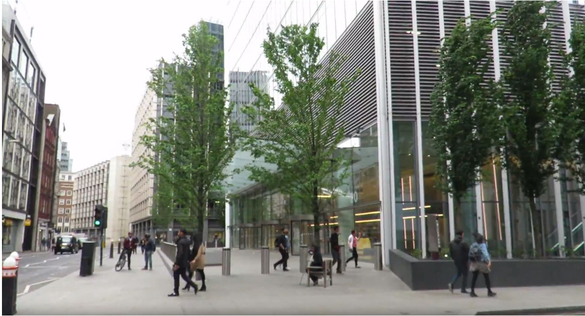
Figure 18 Corner effect. "Walkie Talkie" building, 20 Fenchurch St, London. Proposed trees in a continuous row 10m tall, recommended by wind tunnel testing to reduce dangerous winds at this corner, were never planted. The trees are too far apart and not underplanted as recommended
