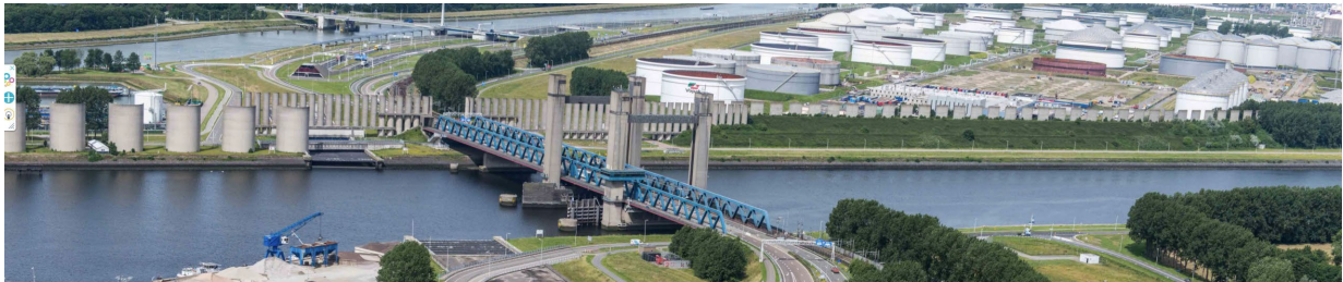
Figure 50 Rozenburg wind wall in Rozenburg, Netherlands, eases the passage of large cargo ships through the narrow canal. The wall blocks about 75% of the of the wind. It is 1600 meters long and is made up of 125 rectangular and cylindrical slabs, each about 25 meters tall and 18 meters wide. (Source: https://bit.ly/2SKLeCG )
