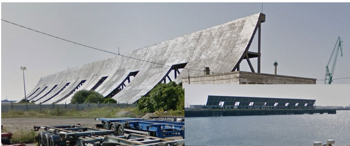
Figure 55 Protection of the boarding quay at Le Havre: concrete springboard ( h = 20\text{ m} , length = 240m) – if this was solid, it is large enough to redirect wind flows
