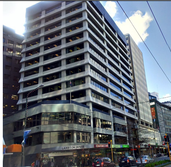
Figure 10 Two buildings with porous facades at car parking levels and with pedestrian level verandahs. Lambton Quay, Wellington
