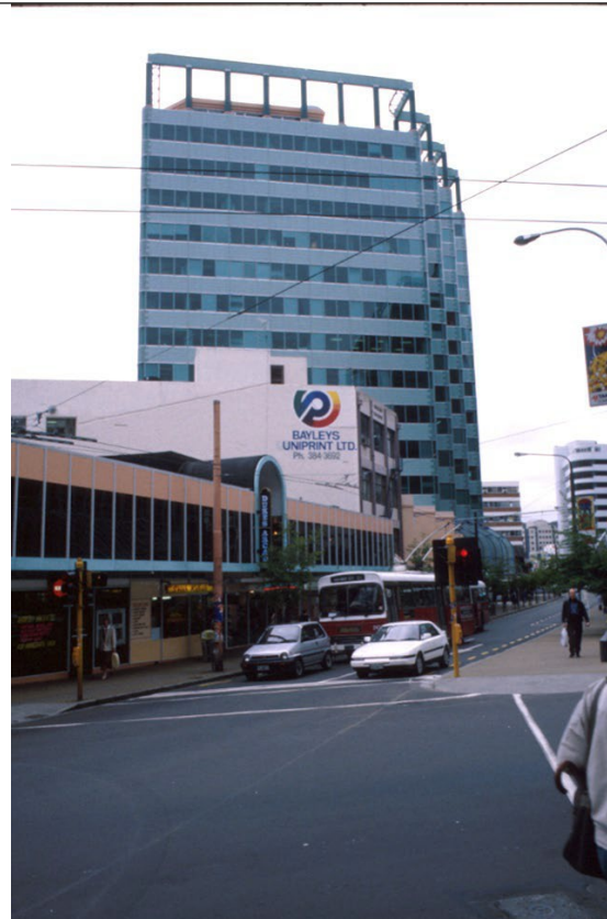
Figure 22 The combination of buildings provides the sort of wind diversion illustrated in Figure 21; Manners St, Wellington
