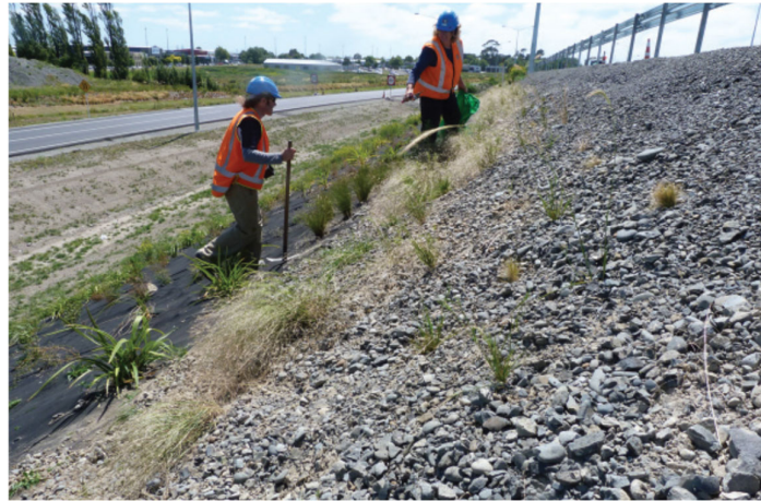
Figure 5. Establishing locally rare native dryland species in a specially prepared stressed niche (very-free-draining exposed substrate) on the Christchurch Southern Motorway extension. Photo: C. Meurk (with permission).
