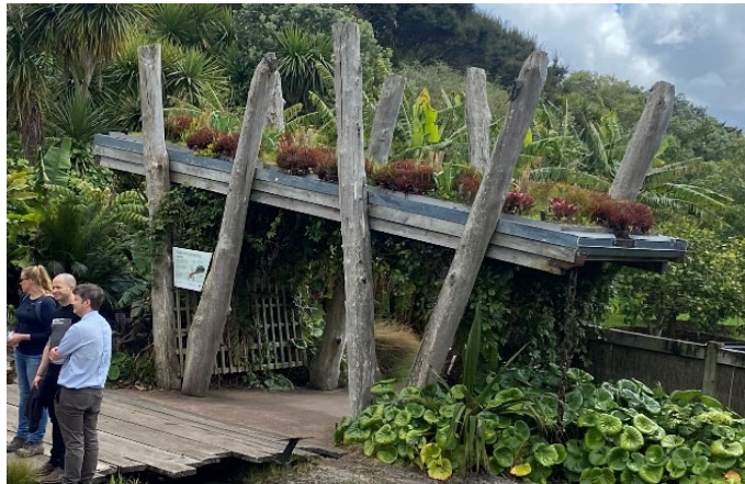
Figure 9. A green roof at the Auckland Botanic Gardens, forming part of the Auckland Sustainable Stormwater Trail. Photo: R. Simcock (with permission).
