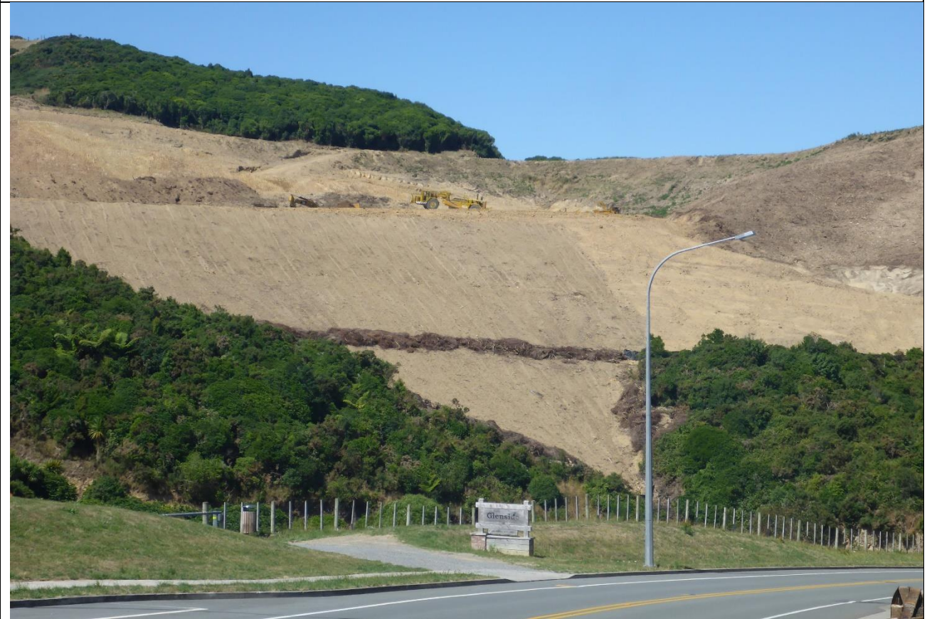
Fig 4C Closeup of earthwork fill slope – Reedy Block Phase 1
