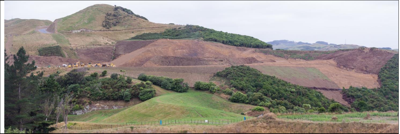
Fig 4B Cut and fill escarpments Reedy Block Phase 1
