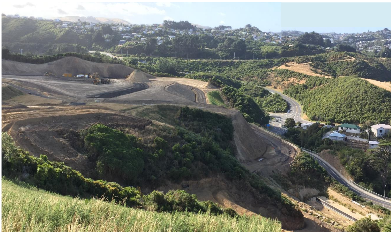
Fig 4A Conversion of natural forms to large flat areas and steep escarpments – Reedy Block, Phase 3
