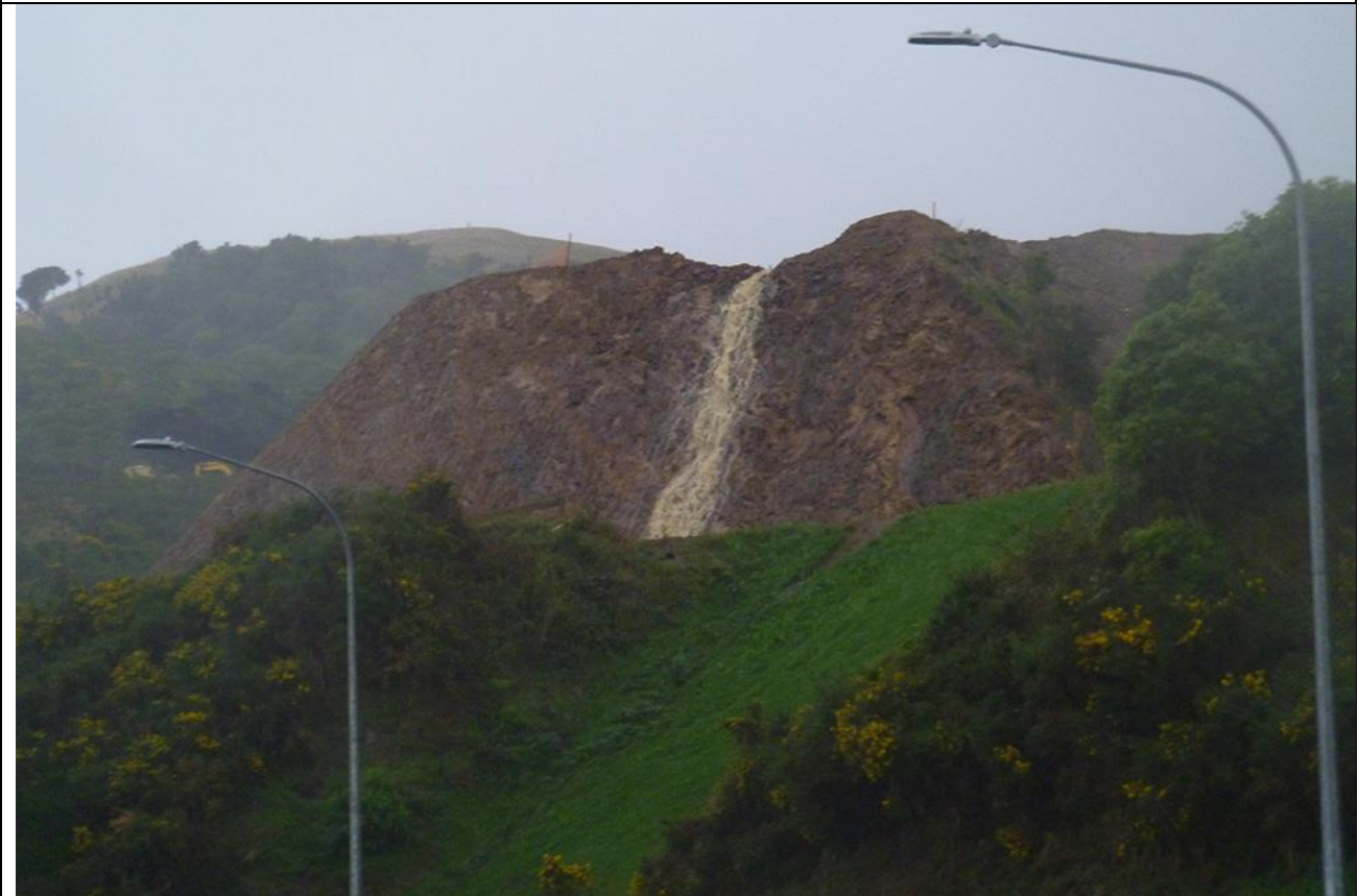
Fig 5 Stormwater runoff from an escarpment within the Reedy Block Development, Phase 2
