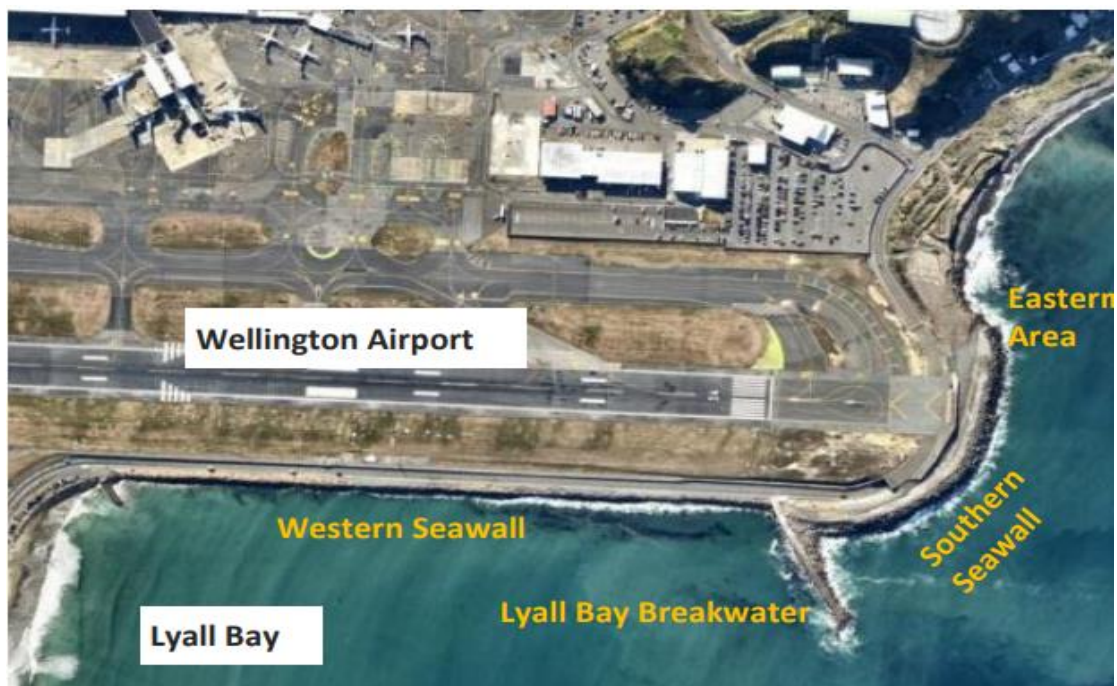
Figure 1: Seawall Structures Lyall Bay
