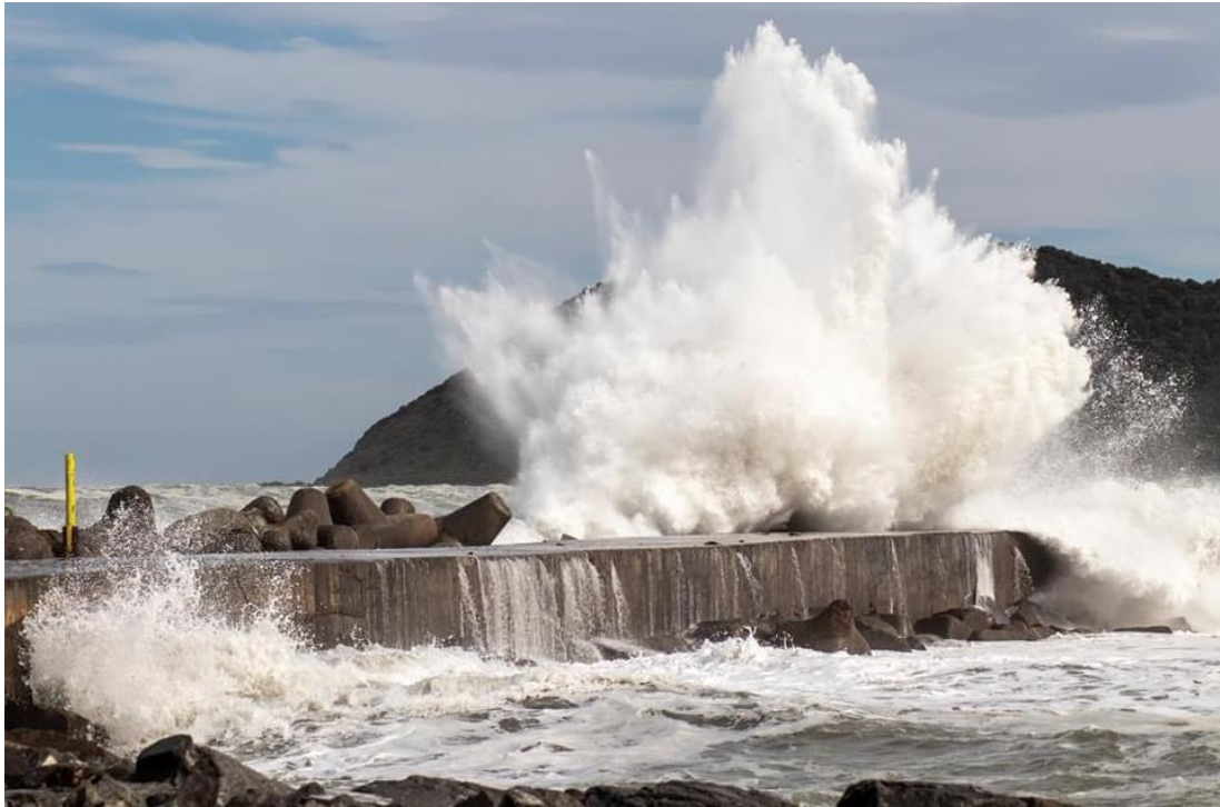
Photo 6: Lyall Bay Breakwater
