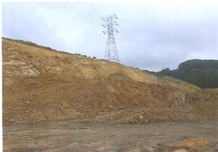
Figure 1: Earthworks in Porirua
