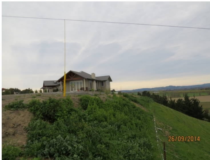
Figure 3: Hastings ground clearance violations
