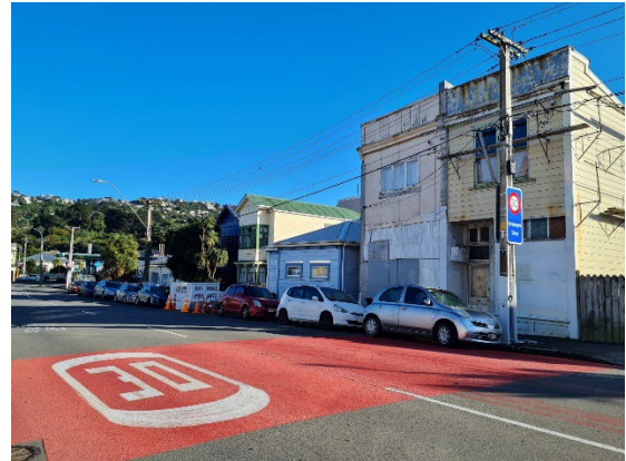
Luxford Street – Looking west from Rintoul Street
