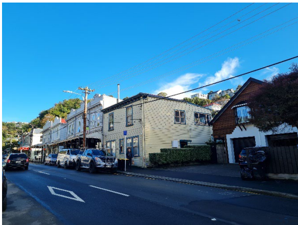
Established centres activity – Hedge shows edge of 22 metre height zone (access to 84 Aro Street)
