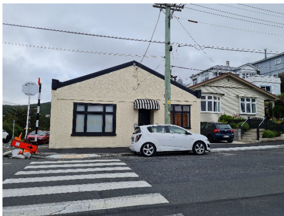
34 Mills Road – Building in residential use
