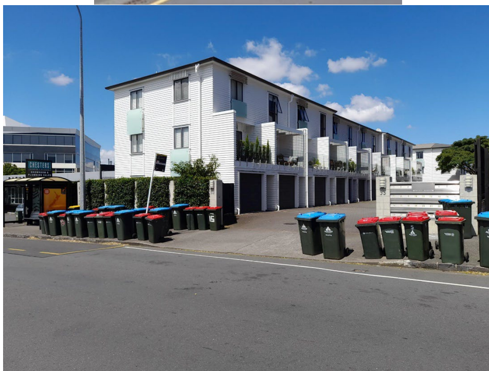
Figure 1 and 2: Multi-unit development bins force pedestrians onto street carriageways.
