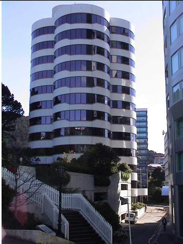
Figure 14 Corner effects of an isolated building are mitigated by 'cloud' plan shape, Bowen Street, Wellington
