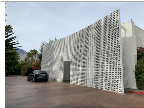
Figure 44: Concrete breeze block shade screen on the Parker Palm Springs Hotel (Source: https://bit.ly/3iGNLSA ). In another context, this could be a wind break with porosity ~50%
