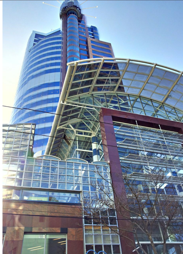
Figure 15 Corner effects of an isolated building are mitigated by the rounded planform, Boulcott Street, Wellington
