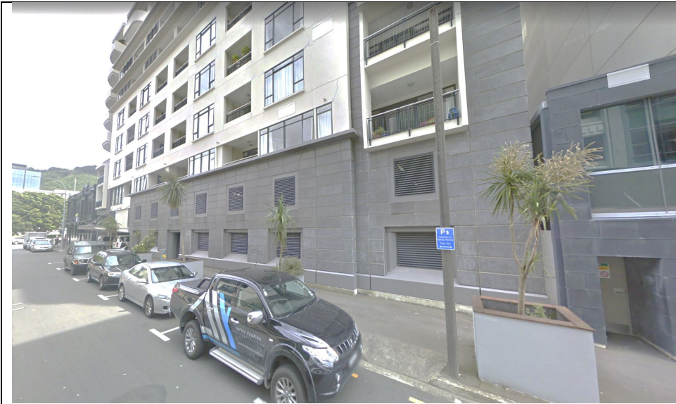
Figure 30 Kate Shepherd Apartments, Wellington, New Zealand. Trees planted by developer as alternative to a canopy wind shelter will never provide the promised shelter, and have become the responsibility of the City Council, not the building owner
