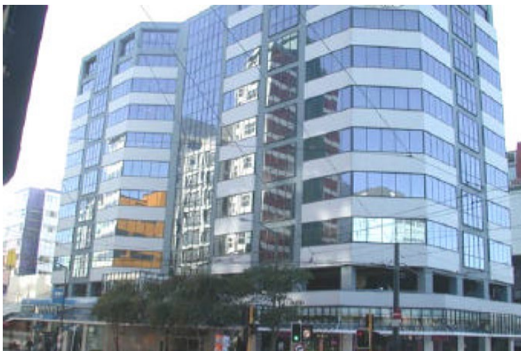
Figure 16 Chamfered corners of the tower reduce the impact on the wind of a broad flat wall, and are simpler to build than a curved planform; also open first floor car parking diverts wind flow above pedestrians. Victoria St, Wellington
