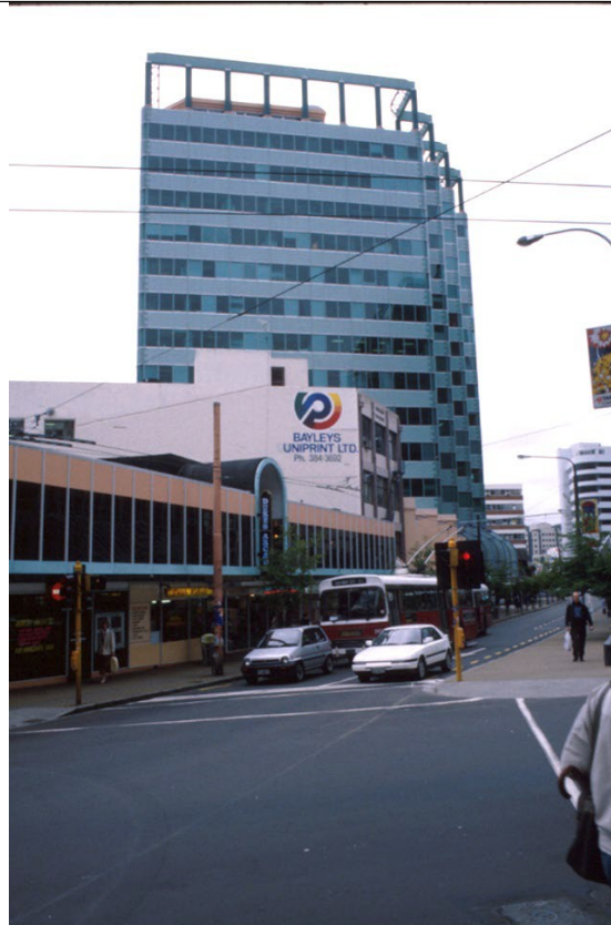
Figure 22 The combination of buildings provides the sort of wind diversion illustrated in Figure 21; Manners St, Wellington
