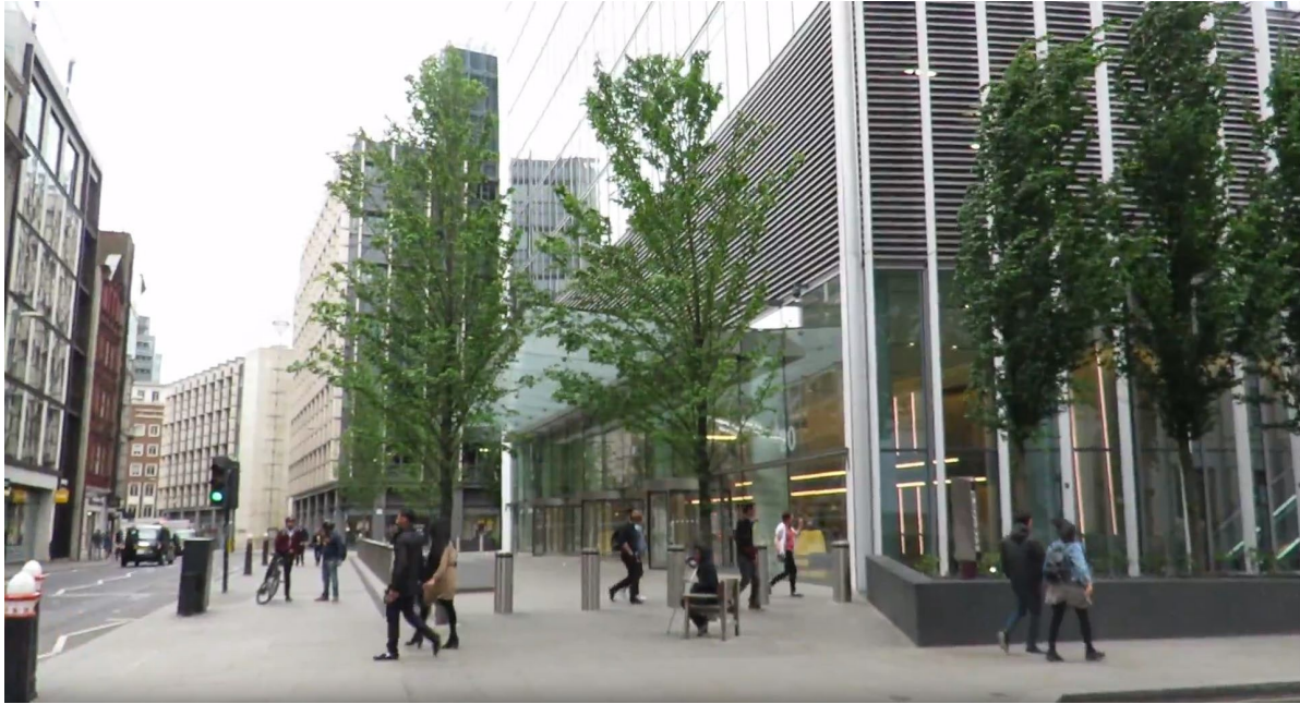
Figure 18 Corner effect. "Walkie Talkie" building, 20 Fenchurch St, London. Proposed trees in a continuous row 10m tall, recommended by wind tunnel testing to reduce dangerous winds at this corner, were never planted. The trees are too far apart and not underplanted as recommended
