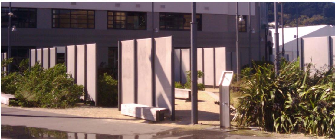
Figure 51 Porous metal screens enabling wind hardy plants to grow beside the harbour in Wellington, New Zealand
