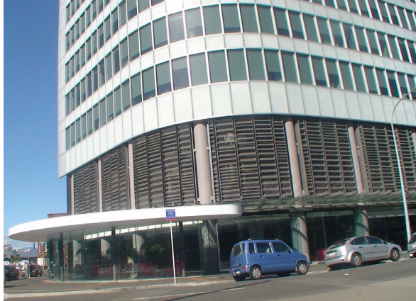
Figure 9 Even with extensive verandahs and a porous façade for the two storey car parking levels above the first floor, the sheer bulk of this building causes significant deterioration in wind conditions on the adjacent footpaths. Featherstone Street, Wellington
