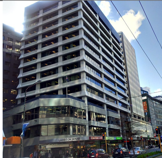
Figure 10 Two buildings with porous facades at car parking levels and with pedestrian level verandahs. Lambton Quay, Wellington
