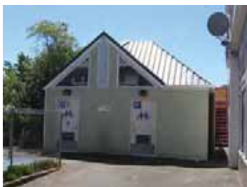
Public toilets, corner Riddiford & Constable Streets
