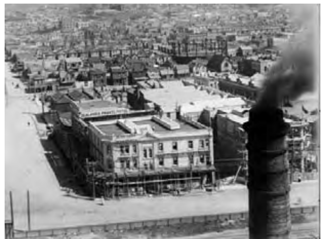
The smokestack of the destructor partially obscures the finishing touches being made to buildings on Wakefield Street in 1908, part of the complete rebuilding undertaken of the former Grainger Street slum. (G019581/1, ATL)
