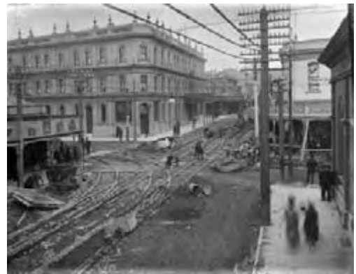
Laying of tracks for the electric tramway, 1903, at the intersection of Manners and Cuba Streets. The still newly constructed Royal Oak is in the immediate background, with the Union Clothing Co. on the other side of the road. (G002130-1/1, ATL)
