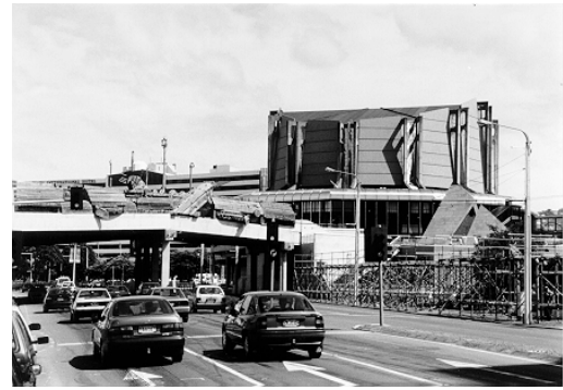
Landmark structures on entrance routes
