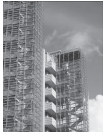
Sophisticated detailing in a contemporary building
