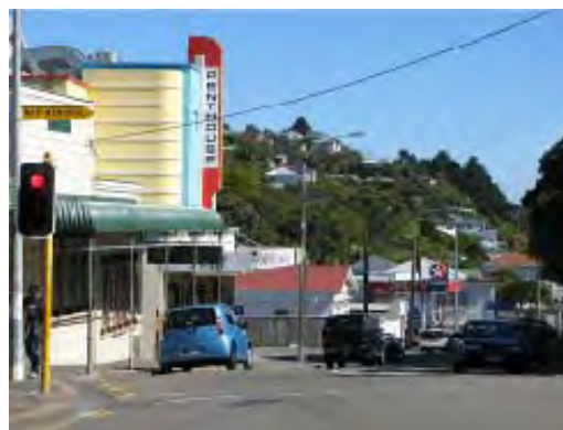
The prominent façade of the Penthouse Cinema is both a local landmark that signals an important community destination
