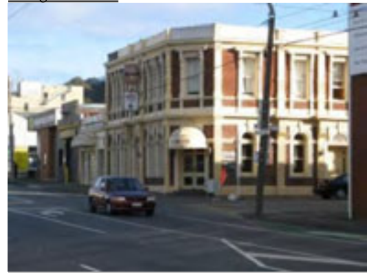
One of the few dispersed heritage buildings, contributing positively to the streetscape
