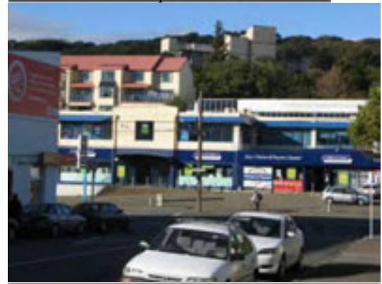
Utilitarian buildings and typical street edge treatment along Adelaide Road
