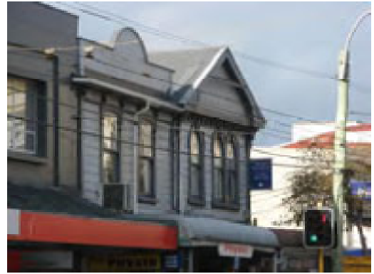
Upper level windows and parapets
