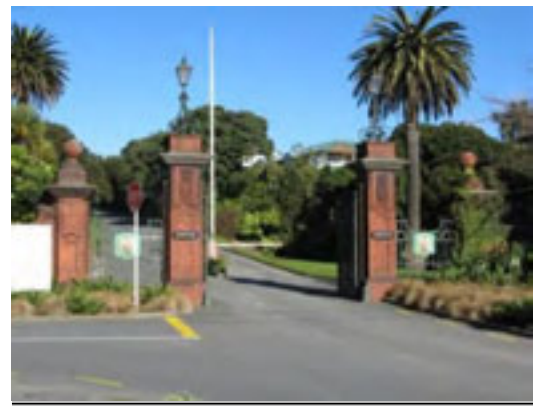
Government House main entrance with related entrance space behind
