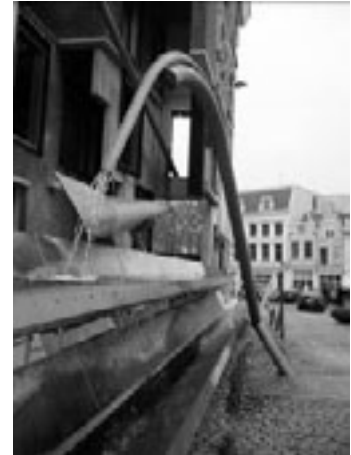
Richness of detail at ground level
