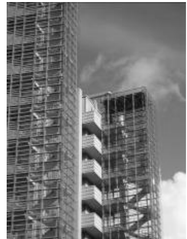
Sophisticated detailing in a contemporary building
