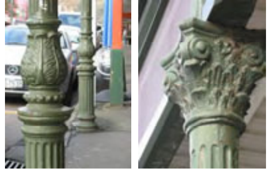
Detail of cast iron veranda posts
