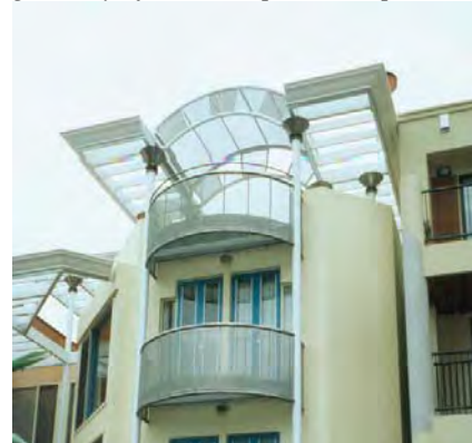
Distinctive building top adds interest to the skyline
