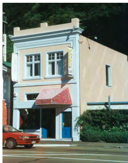
Ground level activities that support the public use of the area
