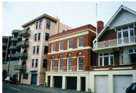
Relationship to heritage buildings is an important design consideration
