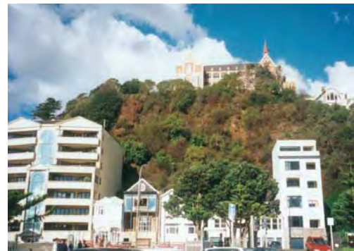
Building tops that project directly against the greenery of the escarpment - a particular concern
