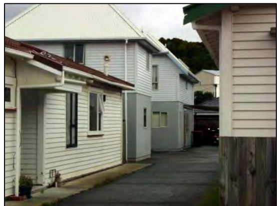
Two additional 2-storey units in the rear yard reduce residential amenity for existing dwelling and adjoining sites.
