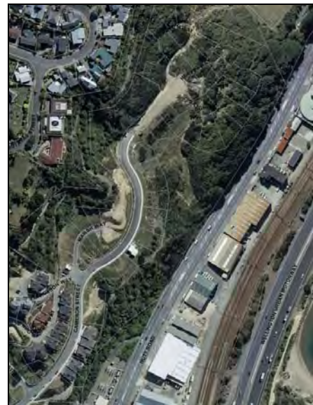
Harbourside development, Kaiwharawhara
