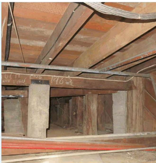
Much of the work is under the floor.
