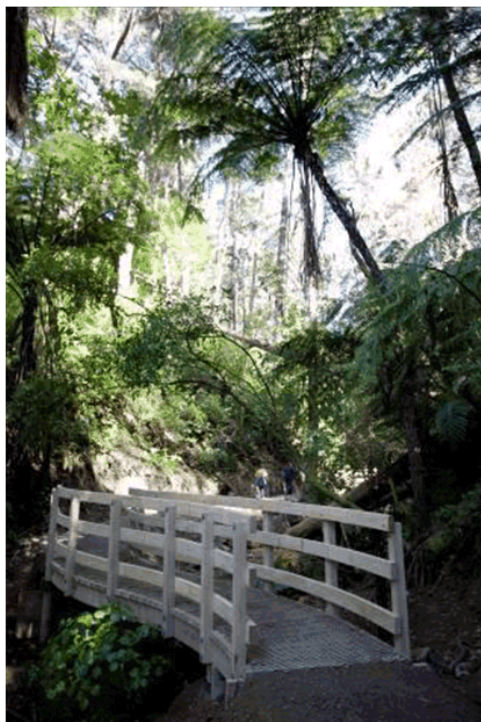
Moturua Stream walkway at Central Park
