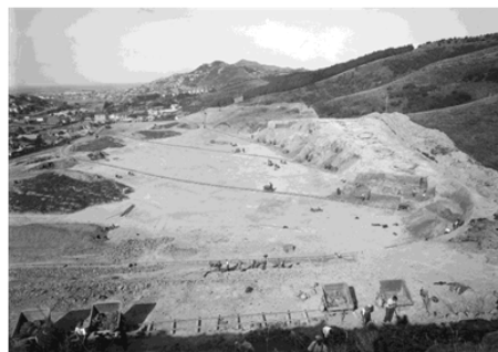
Figure 4: Hataitai Park under construction in 1932. Relief labour dug out banks and moved spoil in metal bins on rails.
