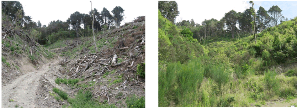
Figure 13: Te Ahumairangi Hill after storm damage in 2004 Left: in 2005. Right: native revegetation 5 years later (in 2010)
