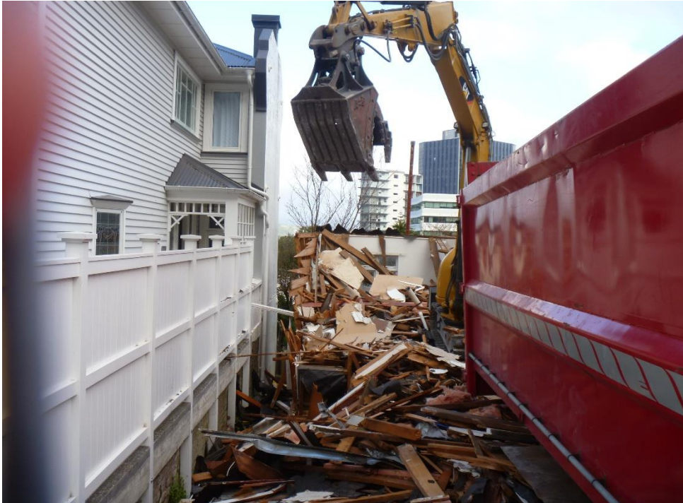
Demolition, Grant Road 2020
