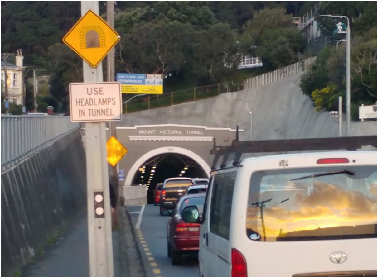
Mt. Victoria Tunnel. Wellington, New Zealand.
