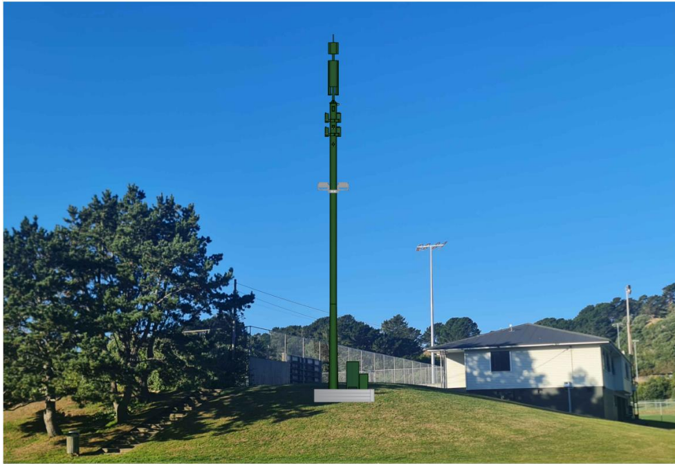
Figure 2. View from sportsfield of the proposed pole, antennas, cabinets and training lights
