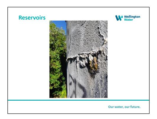
Only two reservoirs exhibited significant signs of structural stress. Both of these reservoirs are to be investigated to determine rehabilitation and/or renewal options.
