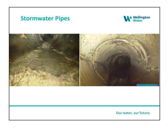
An example of two very poor condition stormwater pipes. As with the reservoirs, maintenance may be possible to maintain level of service rather than renewal.
