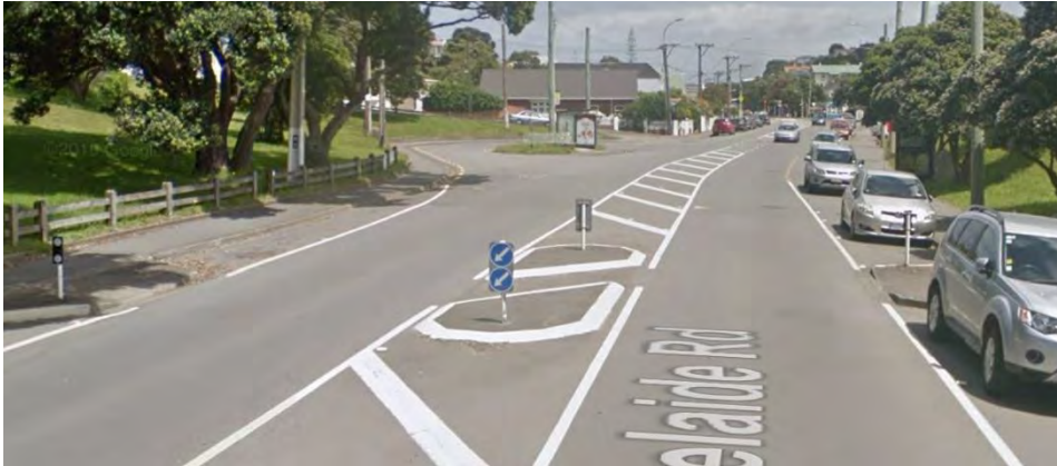
Pedestrian Refuge: Adelaide Road, Island Bay
