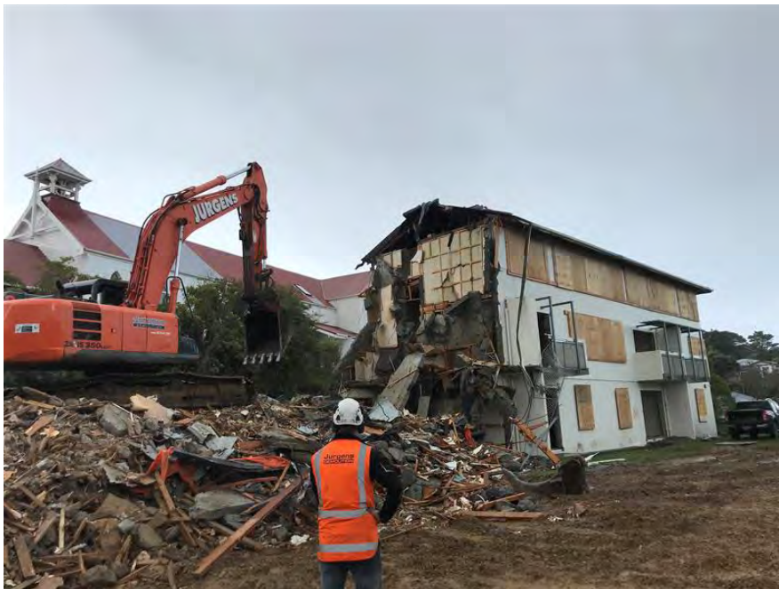
Image 2 – June 2019, midway through the demolition of the old earthquake prone building.
