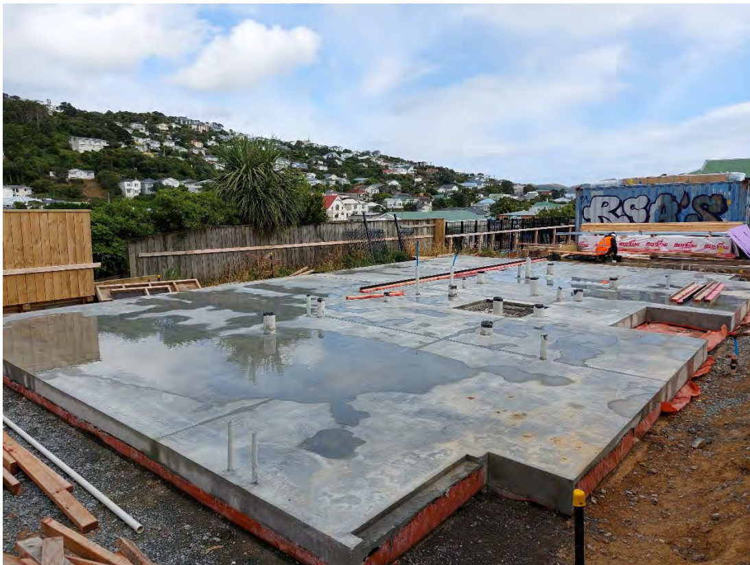
Image 4 – concrete foundations for one of four blocks in the development.
