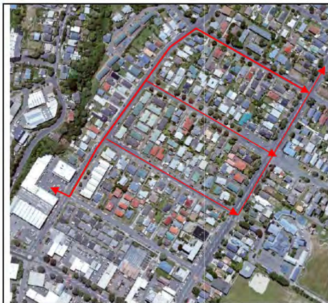
Good access to Tauhinu Road
