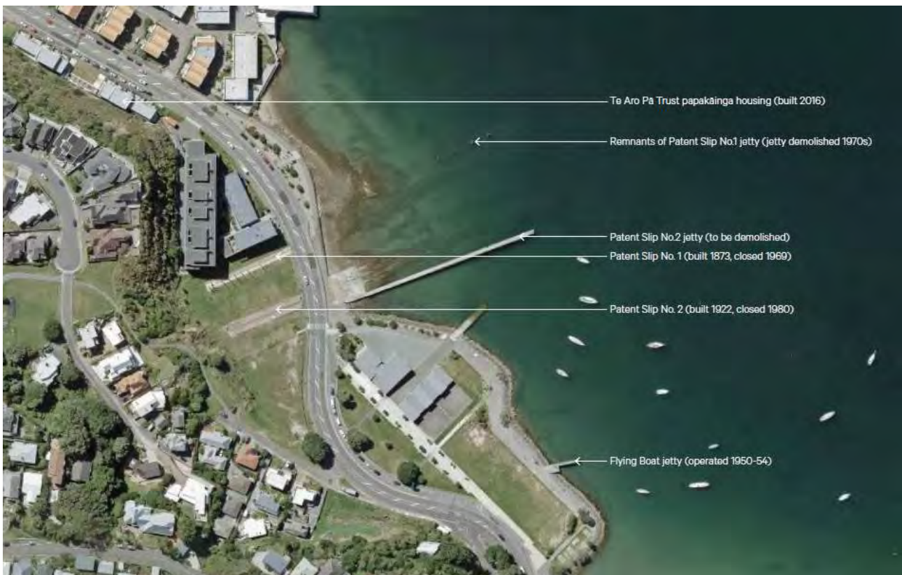
Figure 7: Aerial imagery of patent slip area
