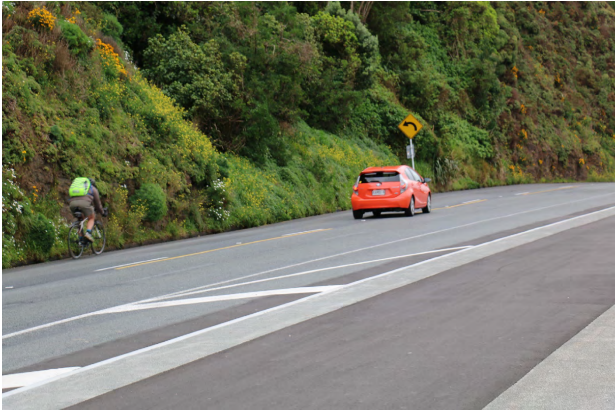
Another car crossing the center line that did not have to before road narrowing changes.
