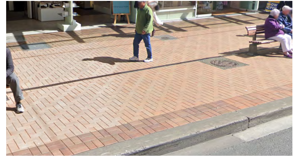
Wider sections of Lambton Quay are in good condition (eg Farmers, David Jones) and support bus stops. Kerbs have a large format profile that lifts the sense of quality.
