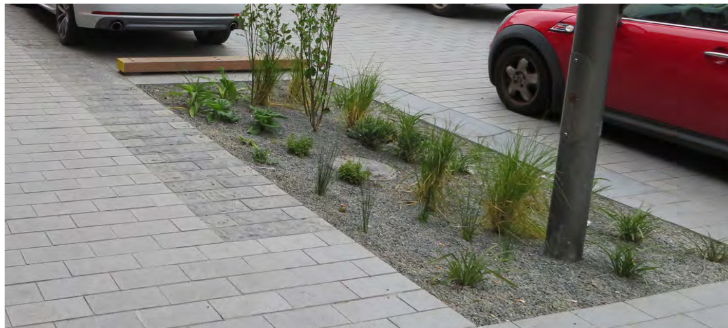
Lombard Lane, Wellington Low growing native planting in raingardens within parking zone.
