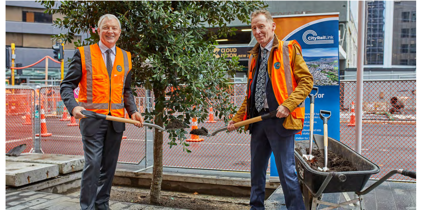
Central Rail Link, Albert and Queen Streets, Auckland Mature native street trees have been successfully transplanted into the central city
