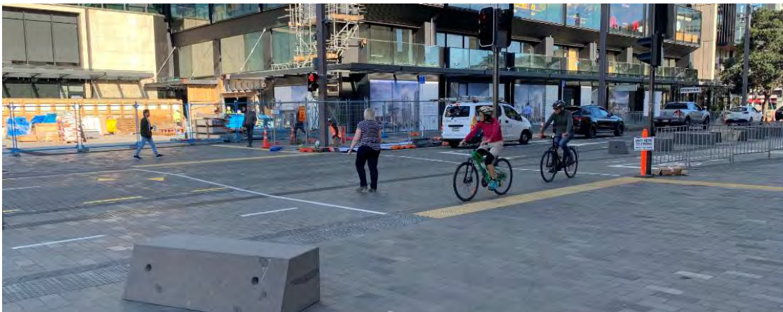
Figure 4-10: Quay Street cycle and pedestrian interface, Auckland
