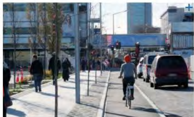
One-way separated cycleway – vertical separation – Colombo Street, Christchurch (photo: Jeanette Ward)
