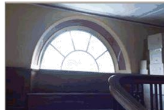
STEEL HALF-MOON WINDOW & TIMBER PANELLING
