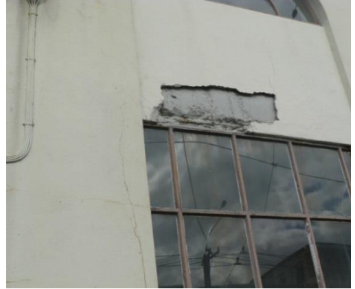
Plaster spalling Sussex St facade
