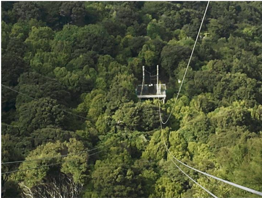
Figure 4: Example of dual ziplines and landing deck.
