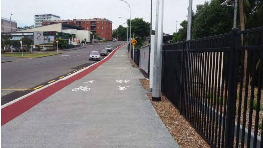
(Above: Shared path with buffer to the kerb, Auckland. Source: NZTA website)
