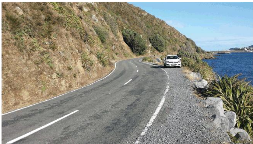
Corner example: steep slope on landward side, some reclamation/strengthening already in place on seaward side (1-2m).
