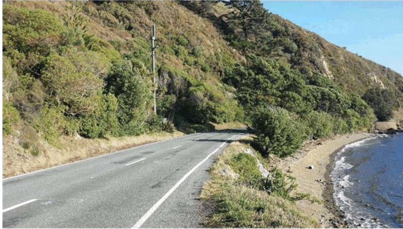
Minimal space between existing service structure and edge of carriageway. Addition of 3m walk/cycle path would effectively remove any beach or recreational area.
