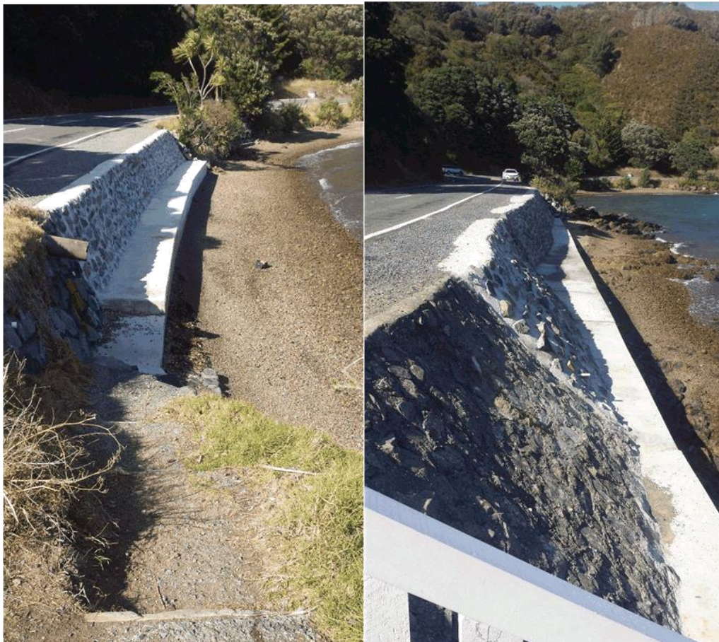
Examples of sporadic reclamations and strengthening works
