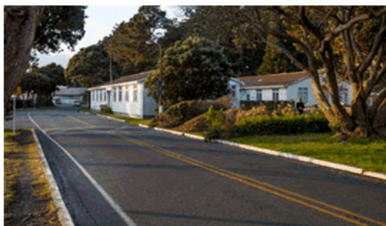
Existing road through Shelly Bay
