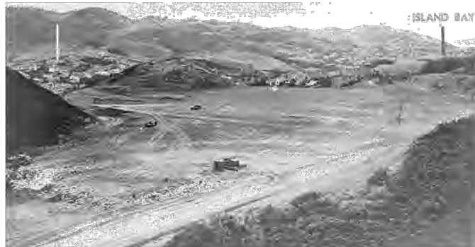
Figure 5: Works in progress, 1949, to transform the Liardet Street tip into a 7 ½ acre playing field - now part of Macalister Park.
