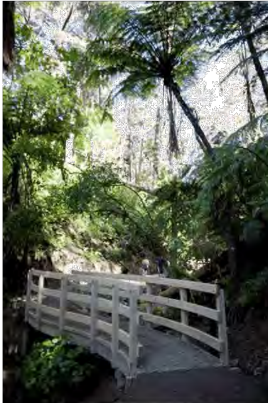
Moturua Stream walkway at Central Park
