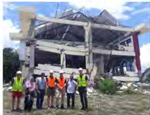
Members of the team assessing a damaged building at Tadulako University. From left: Alejandro Amaris (Miyamoto) Fatmawati Amir (Tadulako University), Prof Iman Satyarno (UGM), Matt Fox, Tony Pettigrew (Beca) Ketut Selandura (Tadulako University) and Andrew Baird (Beca). Rebecca Sanders (Miyamoto) is taking the photo.
