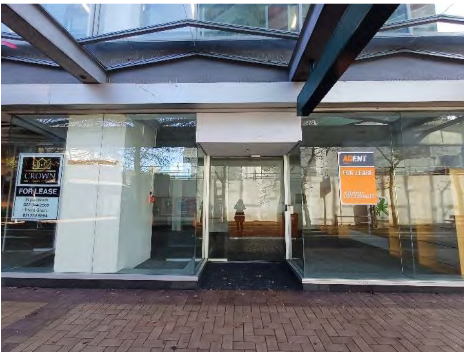
18 Manners Street (below Department of Conservation)
