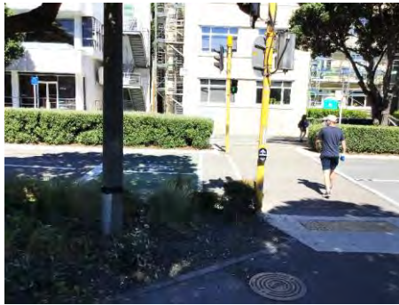
Figure 2-27: Service covers within proposed crossing point
