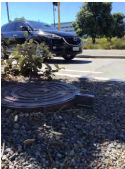
Figure 2-26: Service covers within proposed crossing point
