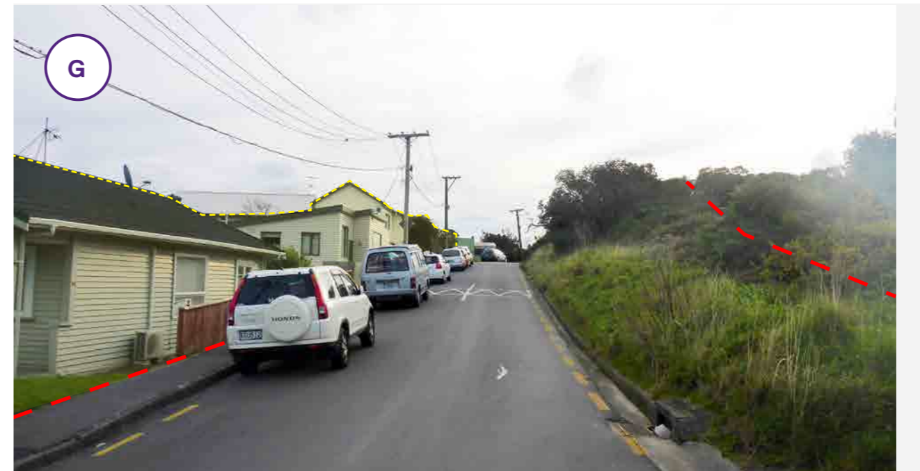
Photo view west along Wexford Road - the airport land is uphill to the right. The dashed red lines show approx road boundary
