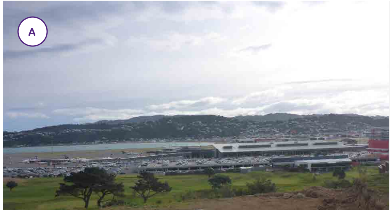
Photo view looking west over to airport from Strathmore area
