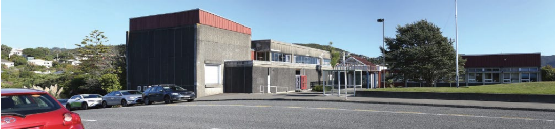
Figure 3: A view from Donald Street showing the Allen Ward Hall (left) and Tennant Block (right) to be retained.
