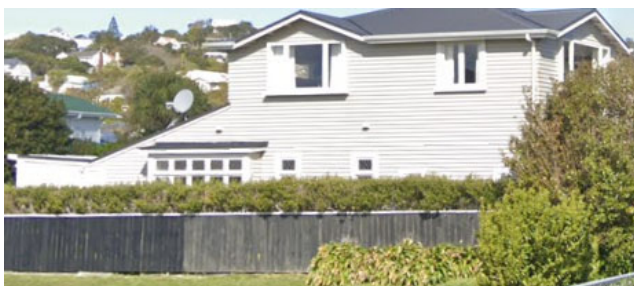
49 Campbell Street, north facade
