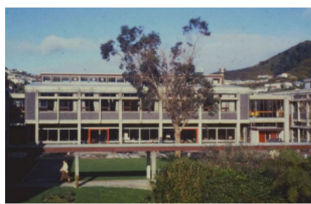
Former Gray & Waghorn buildings
