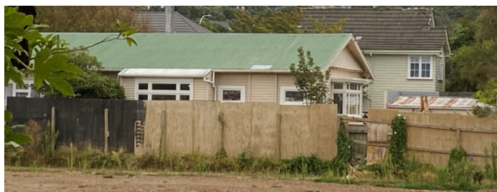
Figure 21: 29 Campbell Street, east boundary with the Site
