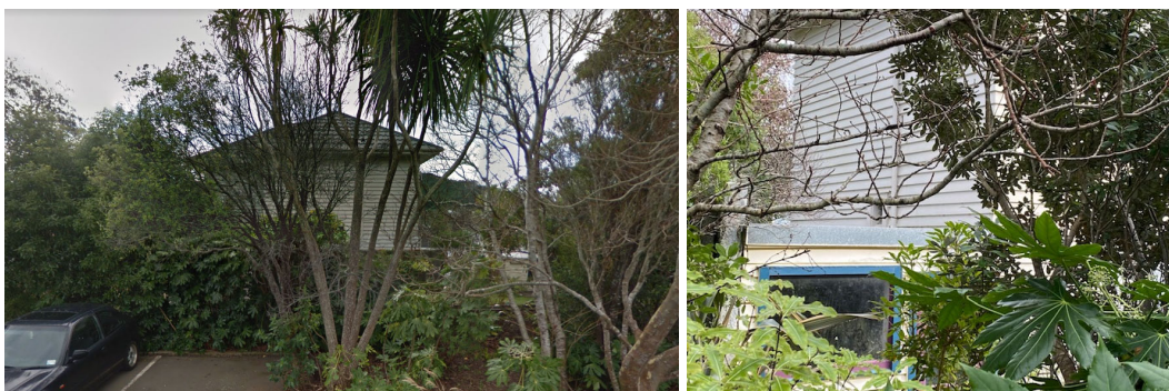
Figure 49: 33A Campbell Street south façade
