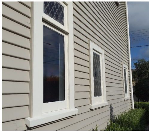
Figure 20: Northern elevation of 49 Campbell Street.
