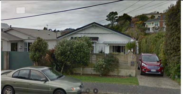
67 CAMPBELL STREET, Karori – House blocked Wall: 0.3m
