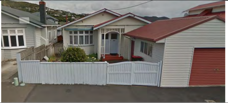
56 Donald Street – House and garage blocked
