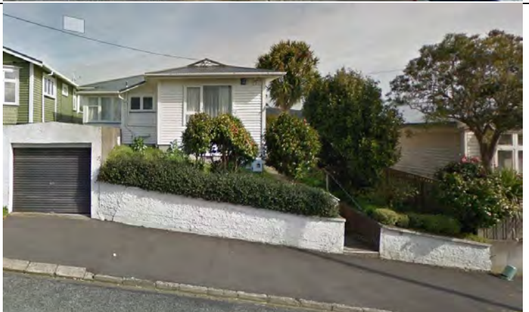
62 Donald Street – House and garage blocked Wall: 0.7m
