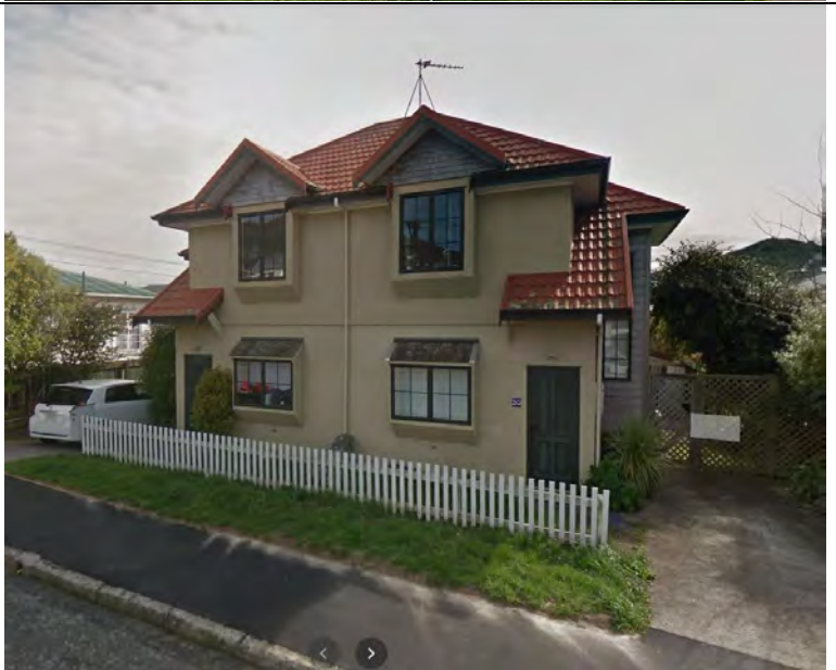
30 - 32 FIRTH TERRACE, Karori, Houses blocked
